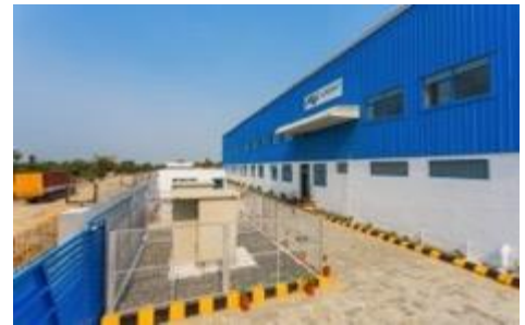
Sipcot Inds Park Chennai Plant
